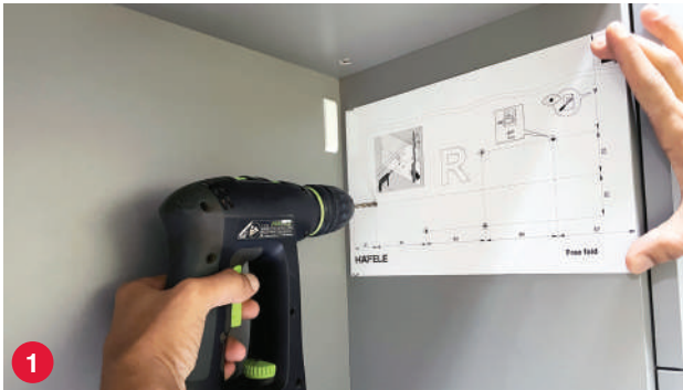
1 DRILLING TEMPLATES: Precise locating of the drill holes is made easier using the paper template provided with each fitting
